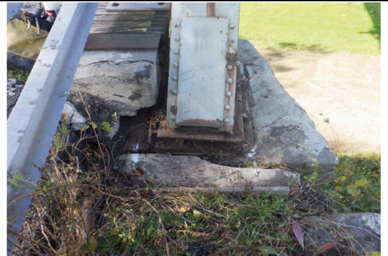
79. General view of the Left Truss bearing at the Far Abutment.
