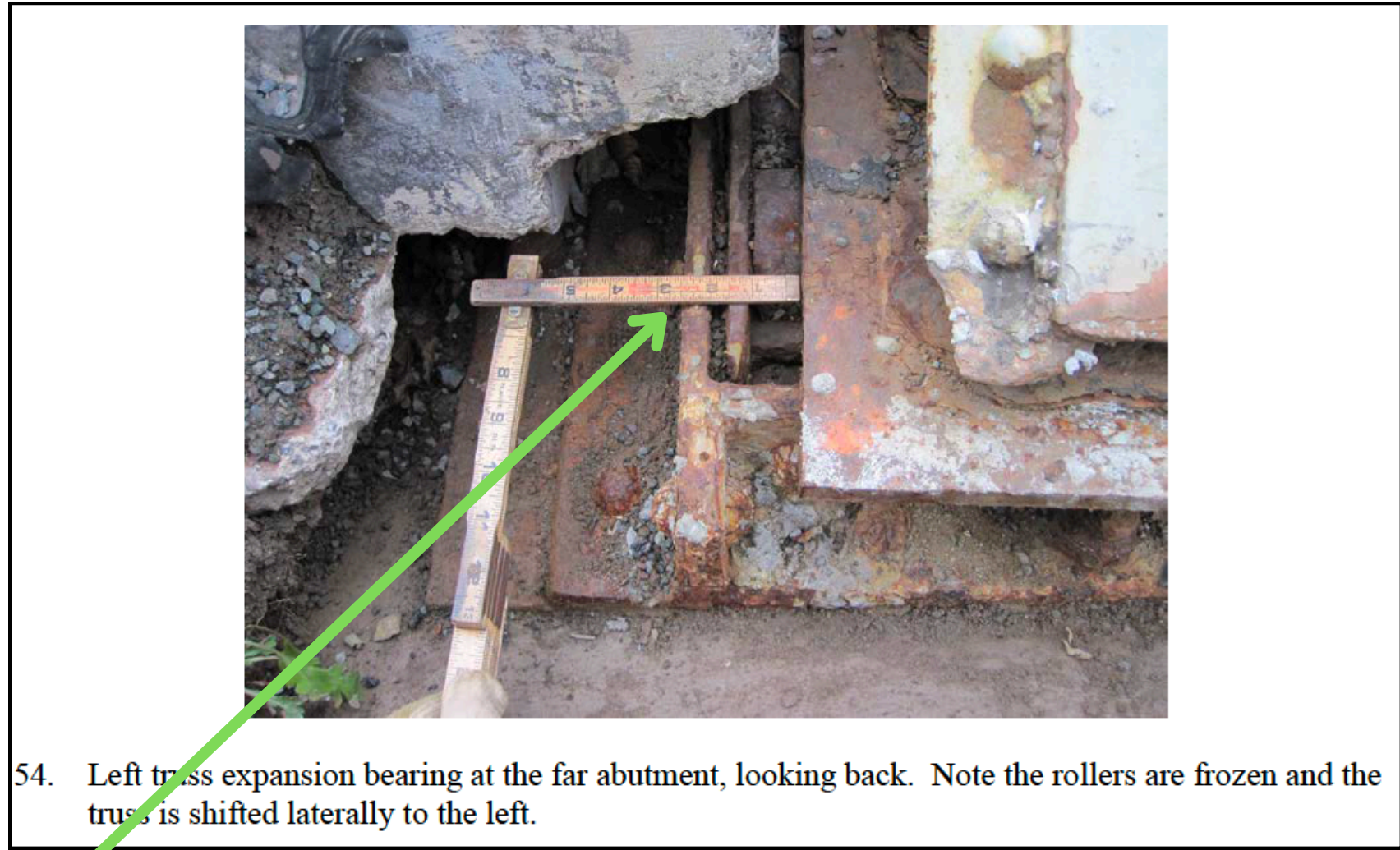
54. Detail of previous photo. Note the truss is shifted laterally to the left and the cap stone is fractured and settled underneath the bearing.
