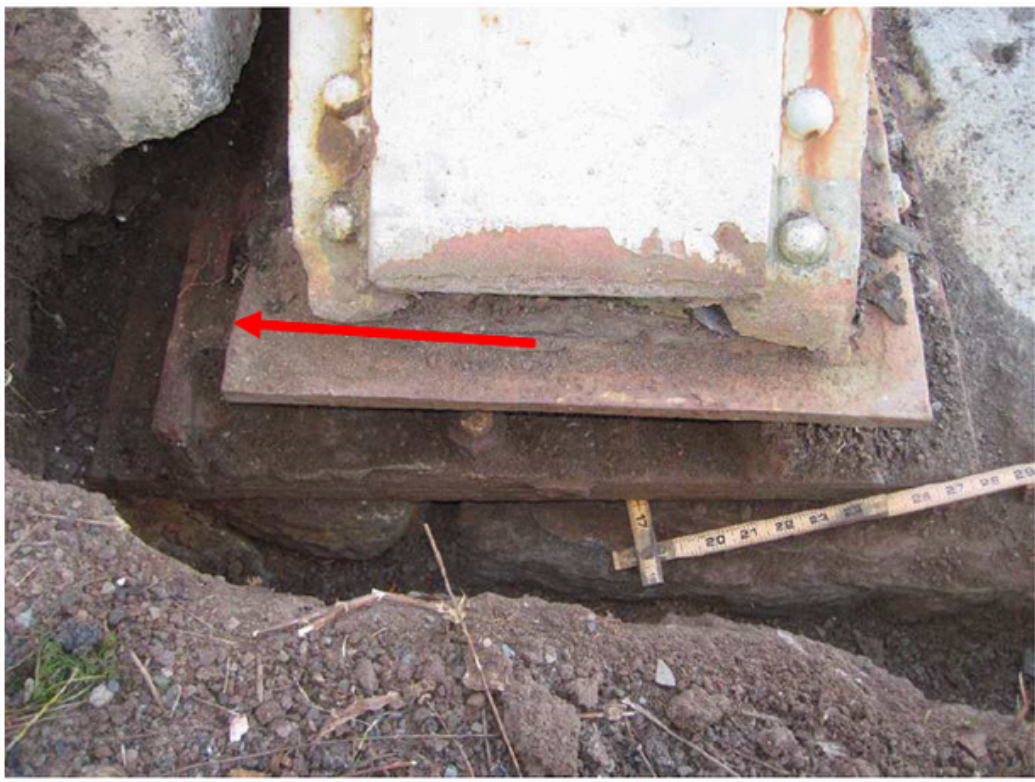
54. Detail of previous photo. Note the truss is shifted laterally to the left and the cap stone is fractured and settled underneath the bearing.
